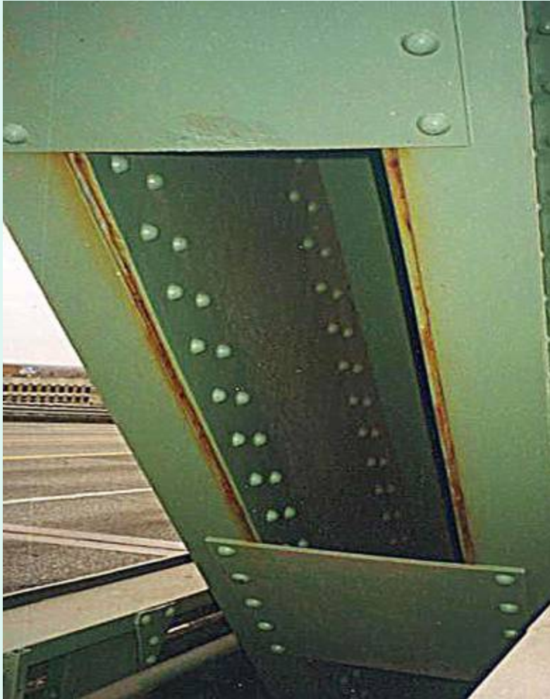
1 yr old 3 coat zinc epoxy urethane over pack rust
